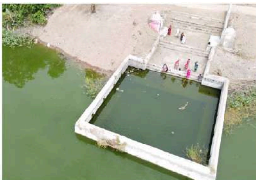
SCARED Vishnupuri Tank – AFTER CLEANING OF DEBRIS & BUSHES
