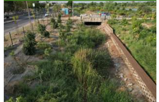
Unification by Hume pipes / culverts. Proposed average water depth after desilting = 2.8 M Proposed water holding capacity = 15.47 Cr. Litres
