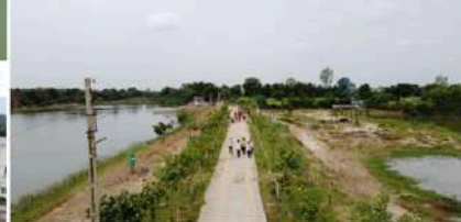
PREPARING FOR AVENUE PLANTATION
