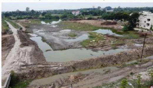
SHALLOW LAKE – DESILTED AND MAKING BUNDS
