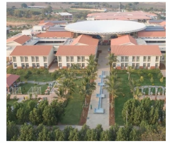
EXTERIOR VIEW OF DORMS (5K CAPACITY)
